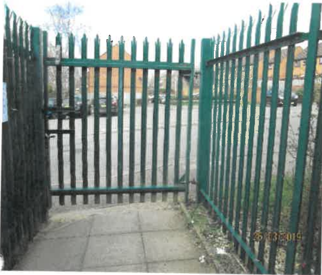
Entrance gate, car parking opposite Centre on Hood Road
