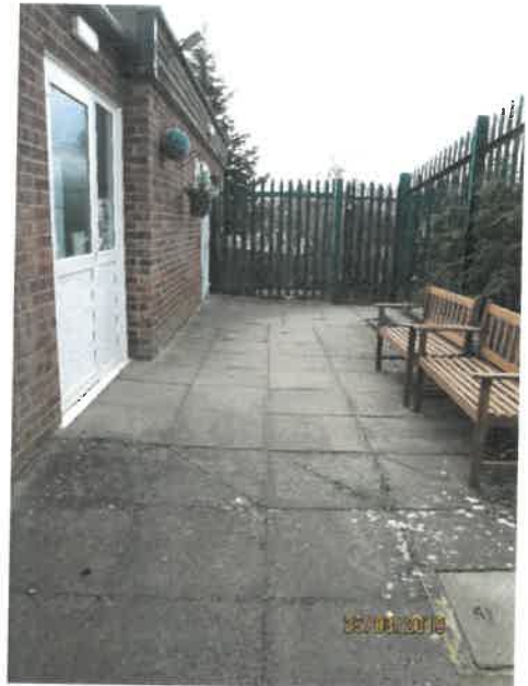
View of front of building Seating Provided.
