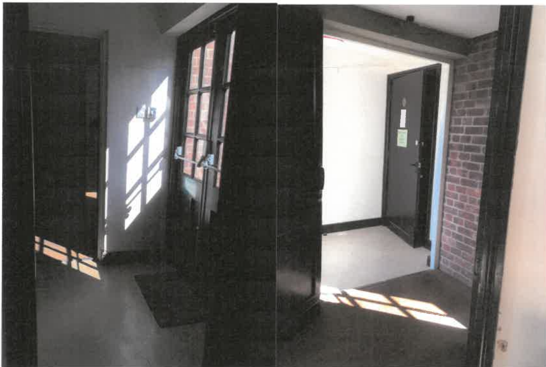
Internal rear access
