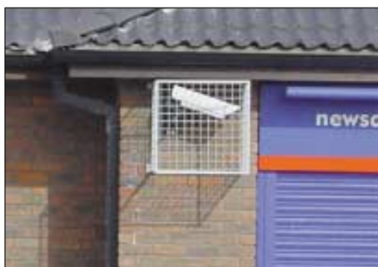
Fig 46: CCTV cameras provide security for a local shop and protect shutters against vandalism and graffiti. Low level camera requires protection against tampering. Source: Northamptonshire Police.
