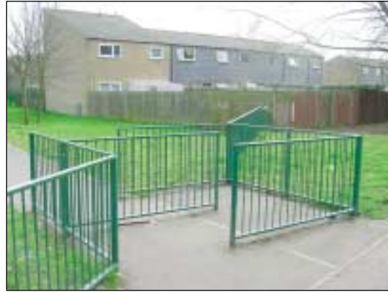
Fig 11: Where appropriate, use gateway features to restrict access by motorcycles. Source: Northamptonshire Police.
