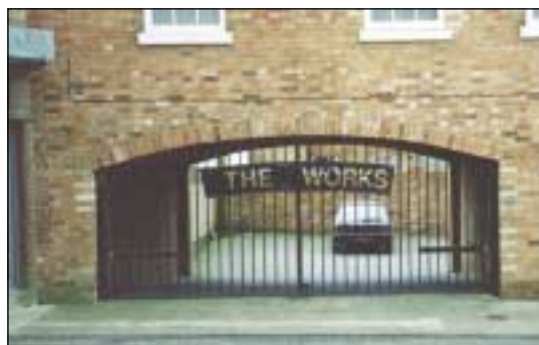
Fig 53: Courtyard parking with secure gated entrance. Source: Northamptonshire County Council.
