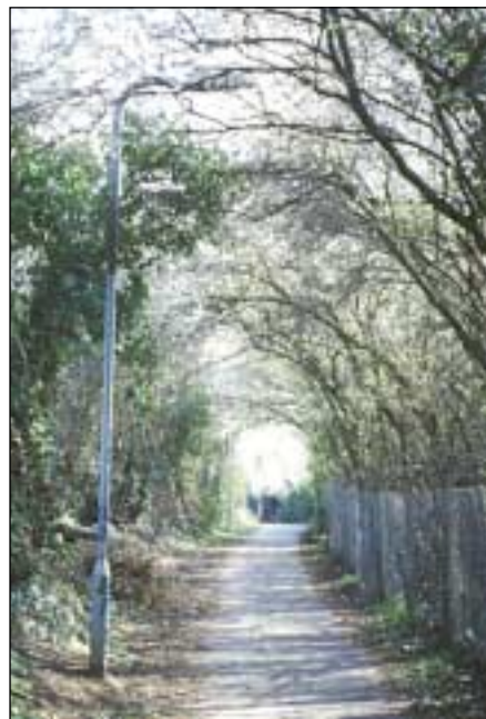
Fig 42: Poor lighting design. Trees reduce effectiveness of lighting and cause shadowing. Distance between lighting columns creates light dark patches. Source: Northamptonshire County Council
