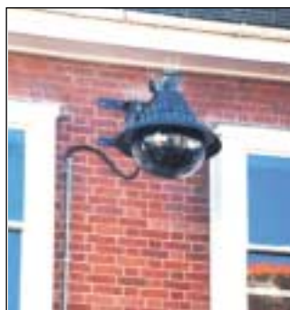
Fig 45: CCTV is more discreetly positioned on the wall of a building. Source: Dudley Metropolitan Borough Council
