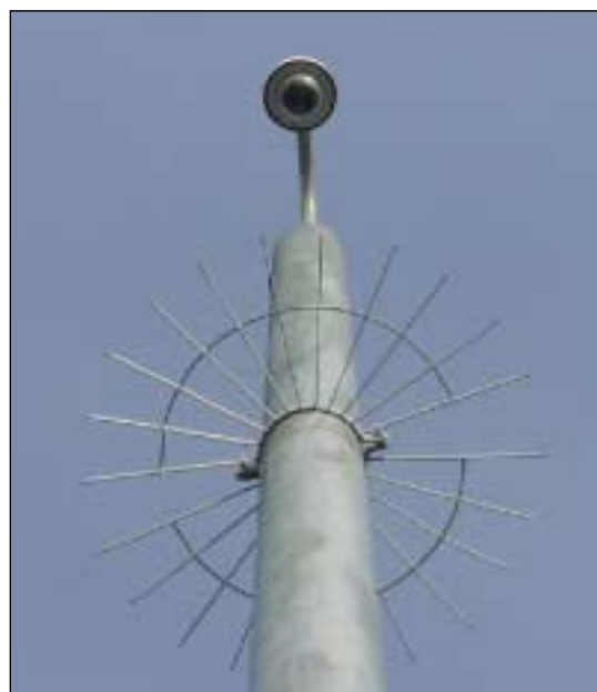
Fig 47: Dome design CCTV prevents detection of the camera’s “eye” direction. A crown of thorns can provide extra security against tampering in high risk areas. Source: Northamptonshire Police.
