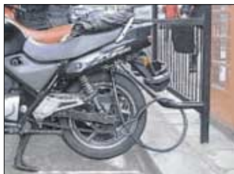
Fig 57: Hitching rail protected by railing to avoid creating a trip hazard to pedestrians. Source: Department for Transport.
