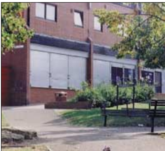
Fig 39: solid shutters create blank and uninviting facade.
