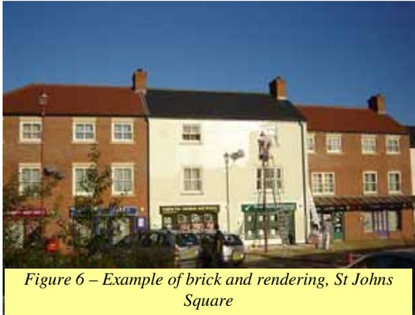
Figure 6 – Example of brick and rendering, St Johns Square
