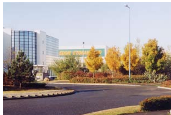
Photo 7: Existing structural landscape
