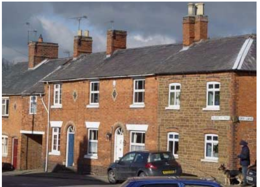
Typical 19 th century brick built, slate roofed cottages in Yelvertoft Road, the right-hand end one stone faced.
